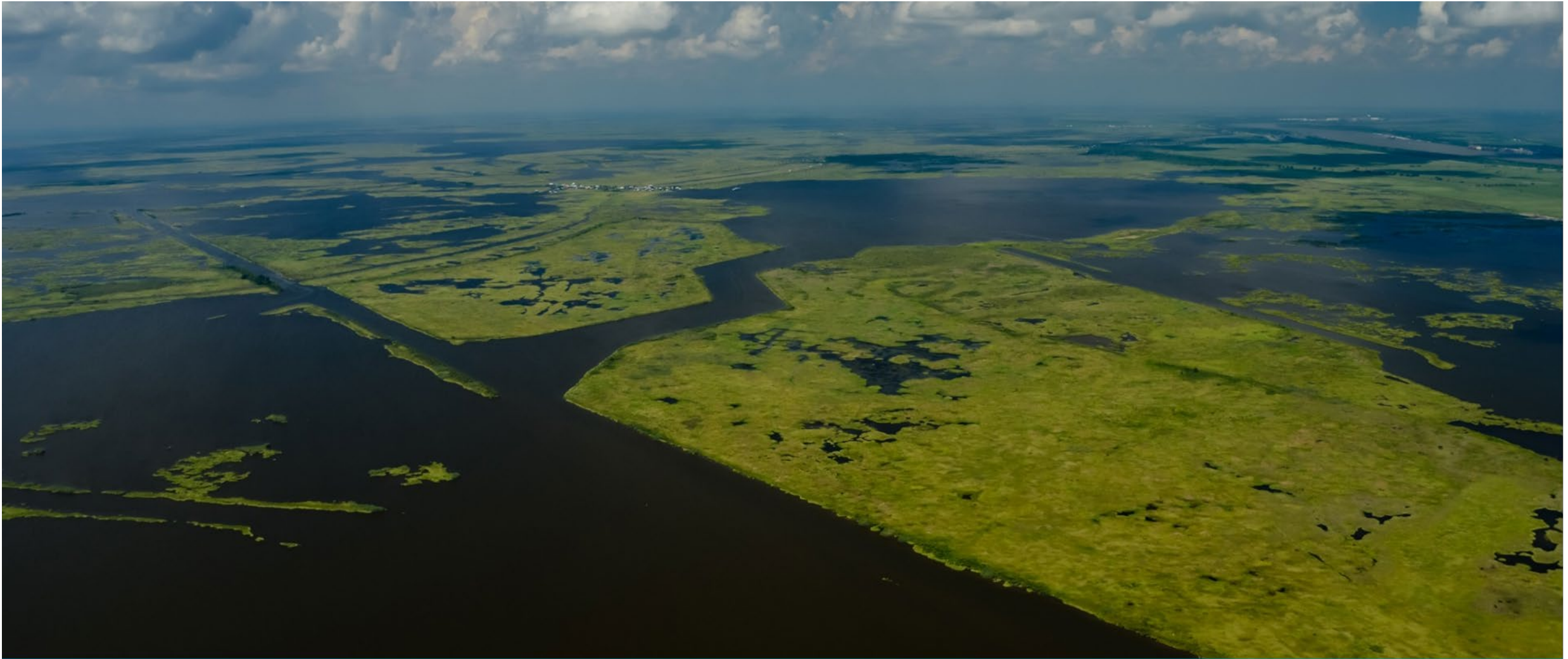
LAKE HERMITAGE MARSH CREATION (CONSTRUCTED IN 2015)
