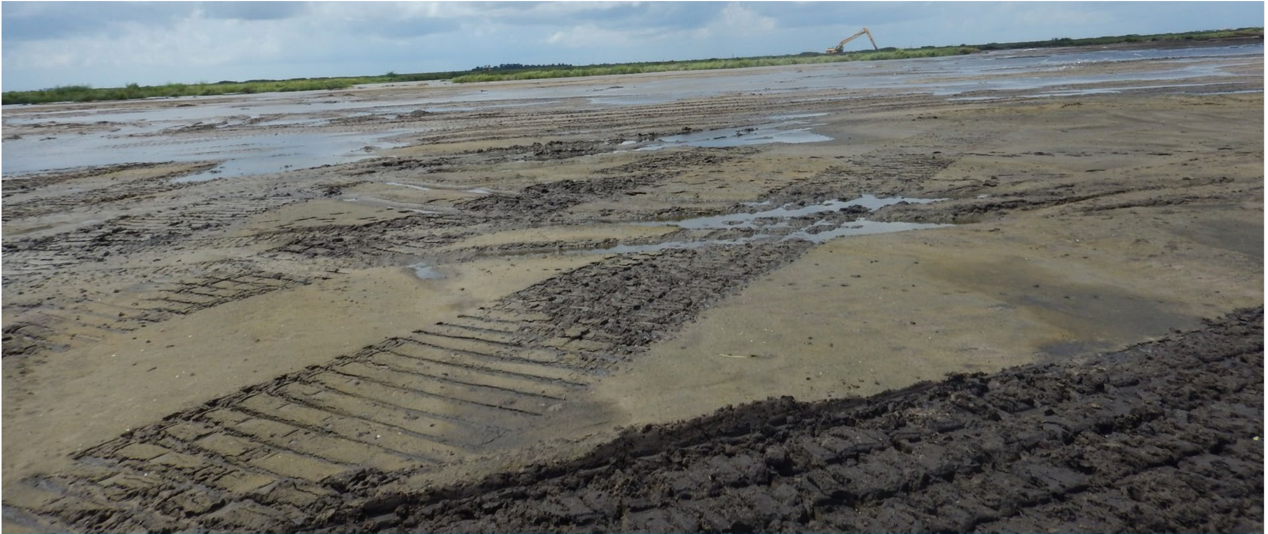
LAKE HERMITAGE MARSH CREATION (CONSTRUCTED IN 2015)
