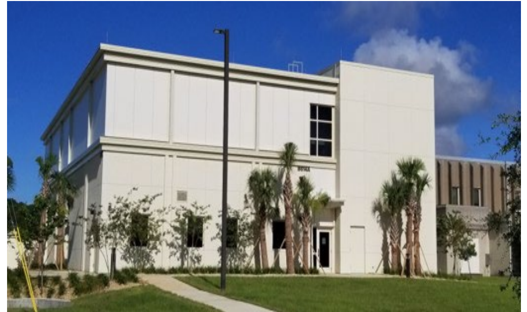
Eglin AFB F35A Armament Research Facility Addition – Small Business Set-aside
